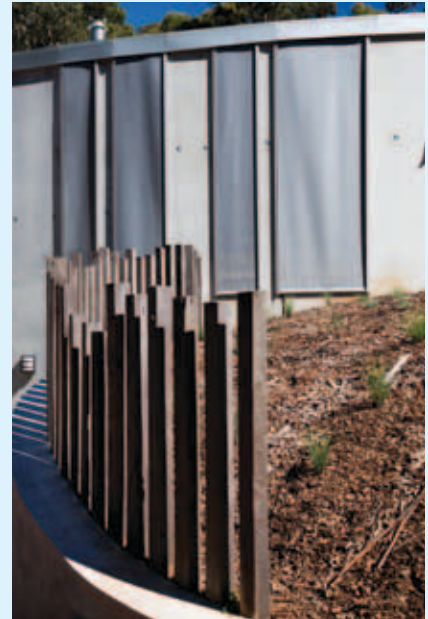
↑ The aluminium frames for the windows and glazed doors were injection-filled with foam to reduce the thermal bridge effect that can be a problem with metal frames. External blinds on all north-facing windows block 95 per cent of the UV light, keeping the house cool and shaded in summer.
